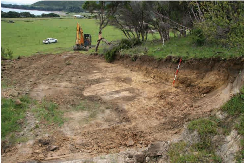
7 (left). Benching works at pole TKH-WAI-A0071 facing east.
