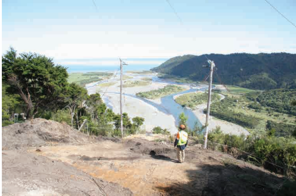
9. Terrace at X15/347 after topsoil stripping, facing north west.
